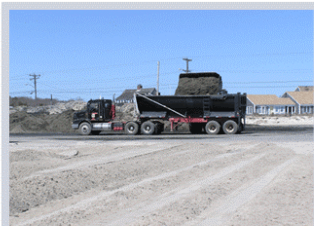
Removal of fine-grained dredge sediment from Craigville Beach to off site locations for beneficial reuse.
